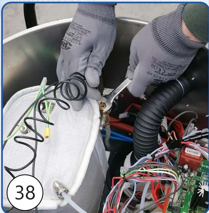
③⑨ Position the bracket on the new boiler, passing the level sensor through the hole.
